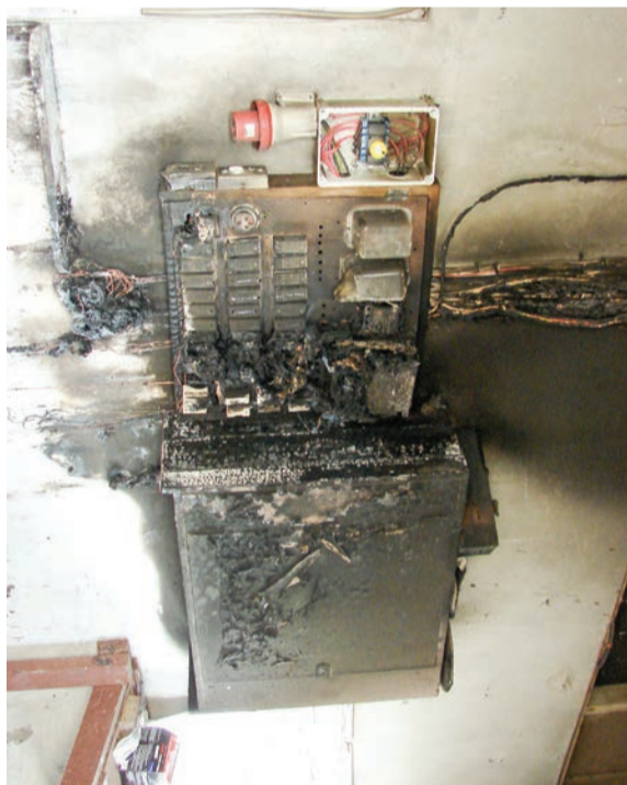
The extensively burnt circuit board.
