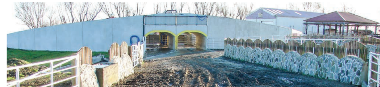
Watino Rock Walls at the entrance to a dairy shed.
